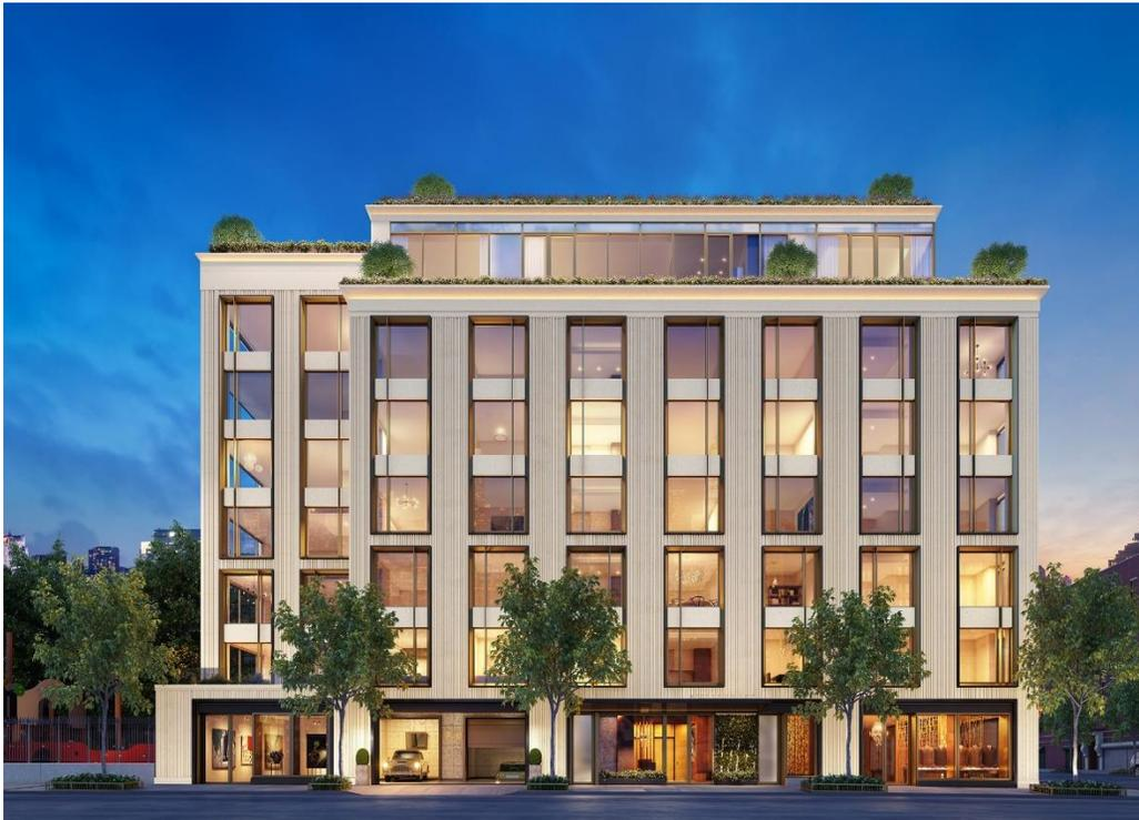
75 Kenmare's façade, designed by Andre Kikoski, is comprised of cast concrete panels and chamfered metal window frames. All renderings courtesy of Redundant Pixel.
